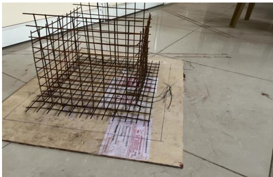
Fig. 3.1: Reinforcement for Foundation and for double wall
