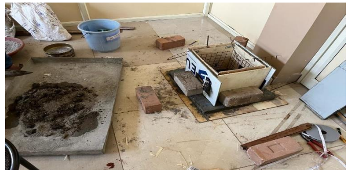
Fig. 3.3: Form Work and Mixing of Concrete
